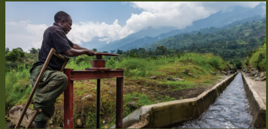
The Mutsora run-of-the-river mini hydroelectric facility is located just outside the Virunga National Park, North Kivu. Photo Credit: Brent Stirton/Getty Images.
